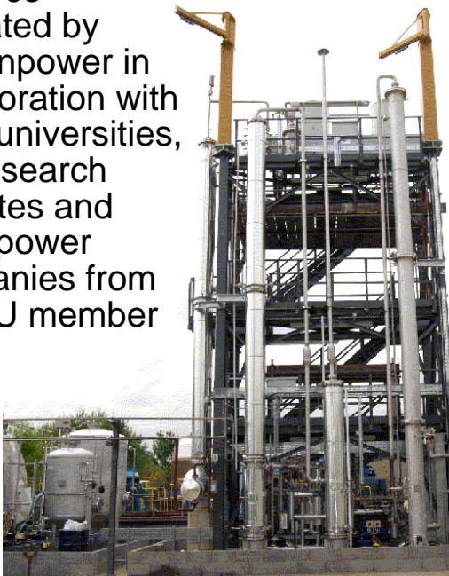
Pilot scale amine test facility
